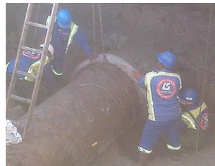
Figure 11: wrapping bidim around the pipe
