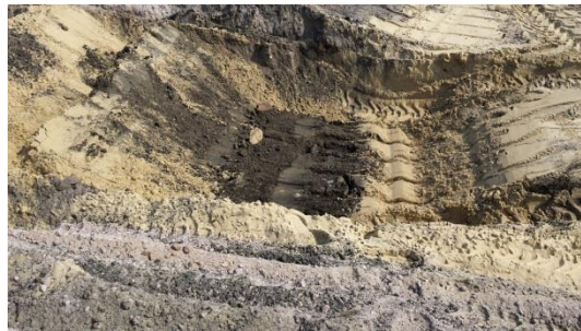
Figure 8: flyash approx 1 meter deep
